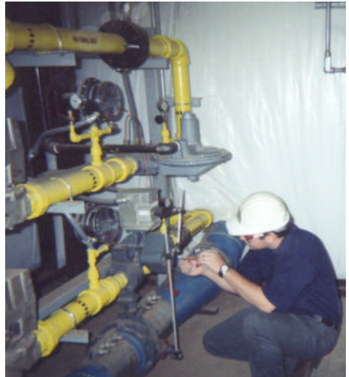
A McGill AirClean field engineer adjusts an RTO gas train.
