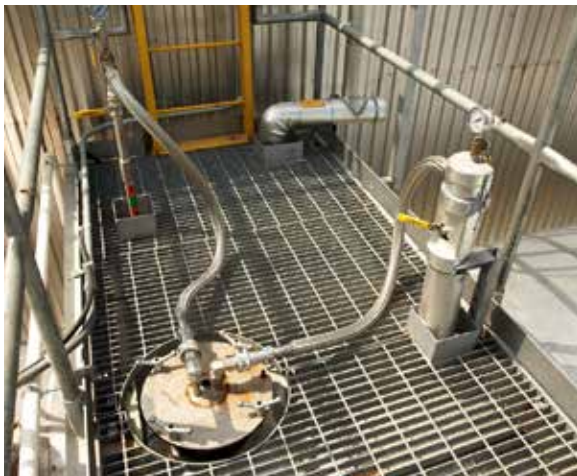
The McGill deNOx reactor uses an injection lance that can either spray the reagent into the flue gas stream as a mist or inject it as a gas.
