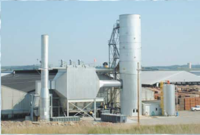
A McGill AirClean Model 3-500 dry EP and spray-dry scrubber control acid gases and particulate from three kilns at a brick manufacturing plant in Ohio.
