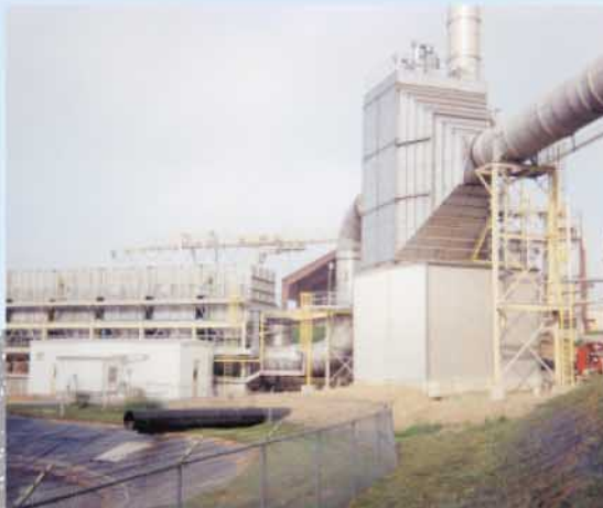
McGill AirClean's ThermoGrid™ regenerative thermal oxidizers (RTOs) control volatile organic compounds (VOCs) for a variety of applications and industries at substantial energy savings over other types of thermal oxidizers.
