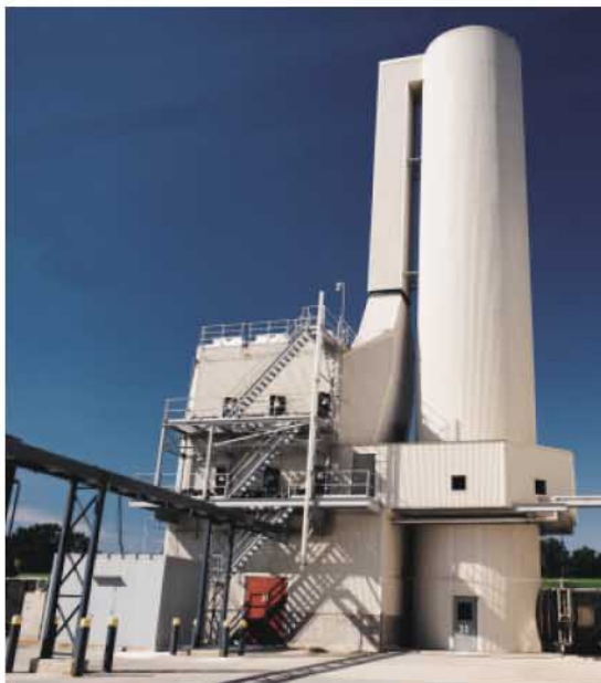
A McGill AirClean spray-dry scrubber and Model 3-500 dry EP collect \text{SO}_x and particulate from the gas stream of a float glass furnace in Wisconsin.
