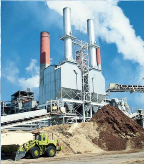
McGill AirClean has numerous installations of dry and wet EPs on wood-fired boilers. The photo on the left is of a Model 3-900 x 2 dry EP collecting fly ash from a paper mill in South Carolina while the photo on the right depicts a Model 3-350 wet EP controlling emissions from a paper mill in Georgia.
