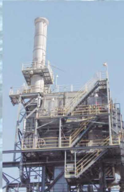
McGill AirClean has numerous installations of dry and wet EPs on wood-fired boilers. The photo on the left is of a Model 3-900 x 2 dry EP collecting fly ash from a paper mill in South Carolina while the photo on the right depicts a Model 3-350 wet EP controlling emissions from a paper mill in Georgia.
