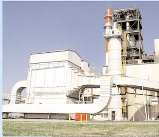
McGill AirClean combined a spray-dry scrubber, dry EP, and two wet EPs to provide air pollution control for this California fiberglass plant.
