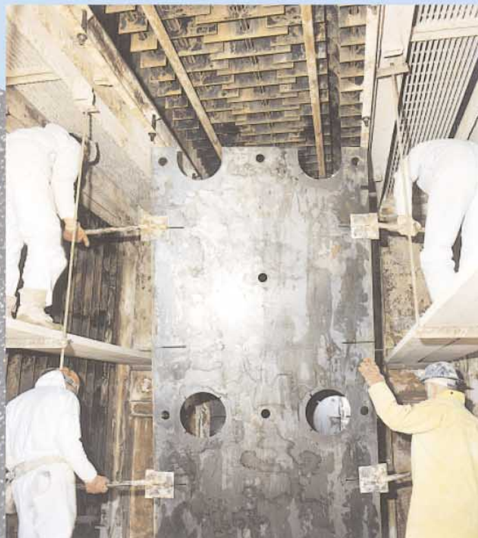
McGill AirClean can rebuild or upgrade older equipment. Technicians here work on a project that included rebuilding the EP's internals and installing a new rapping system.
