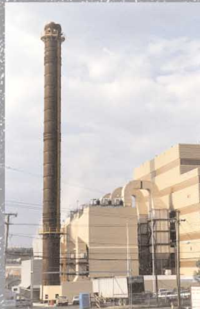
The design, fabrication, and erection of a three-flue exhaust stack, 12 feet in diameter by 210 feet high, was part of this McGill 4-350 x 3 EP system for an Alexandria, Virginia, municipal solid waste facility.
