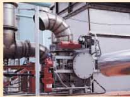
Inlet/outlet duct and connection port for plant's process gas flow
