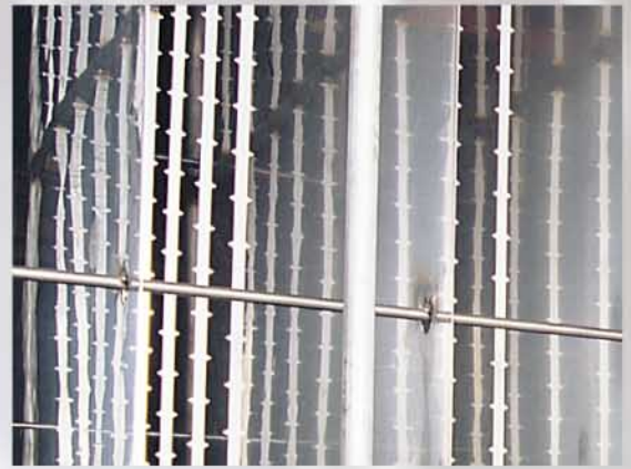
View of the e-frame electrodes and collection plates installed in a module.
